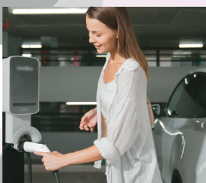
EV CHARGE POINT AT CAR PARKING
